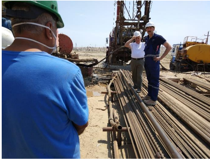
Photo 1. Oil field operation at the Binagadi Oil Company”
